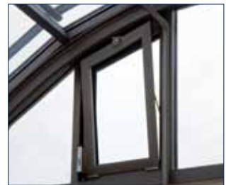
Fanlight opener system with electric linear drive
